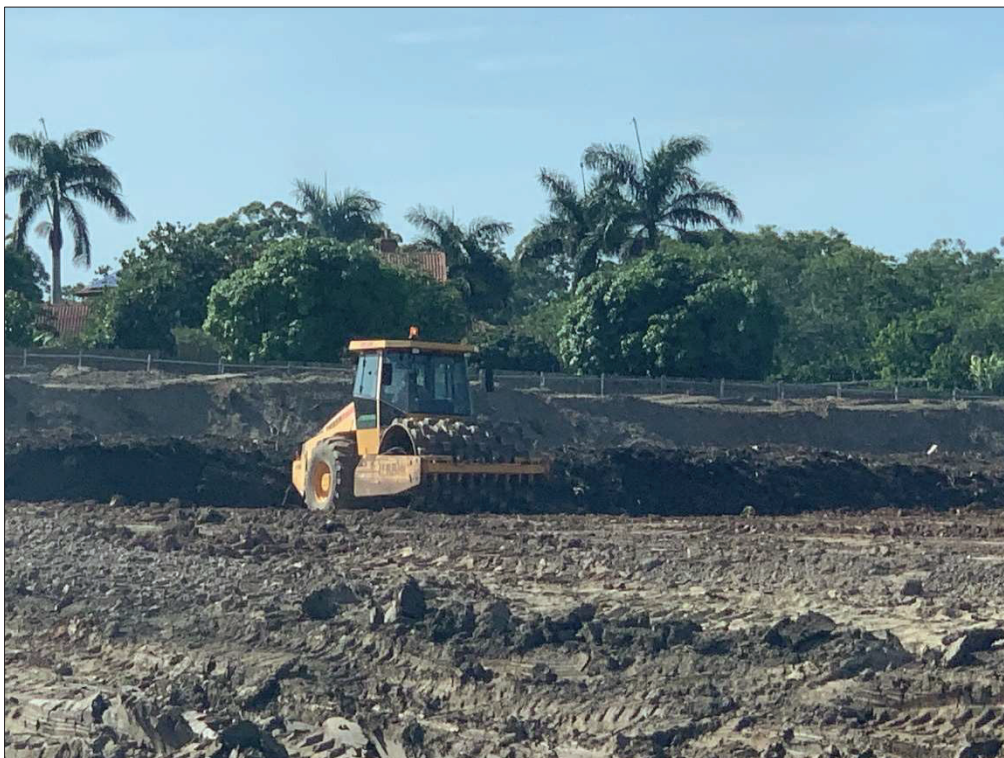
Figure 14. Padfoot roller used throughout earthwork operations to compact material. (Taken 08/03/2021)
