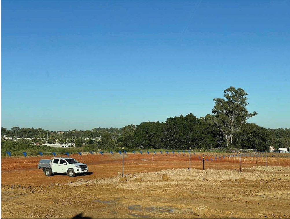
Figure 19. Overview of site. (Taken 21/04/2021)
