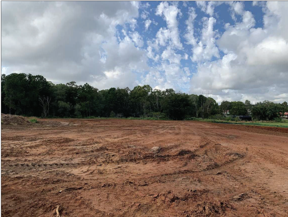
Figure 9. Overview of earthworks pad. (Taken 23/02/2021)
