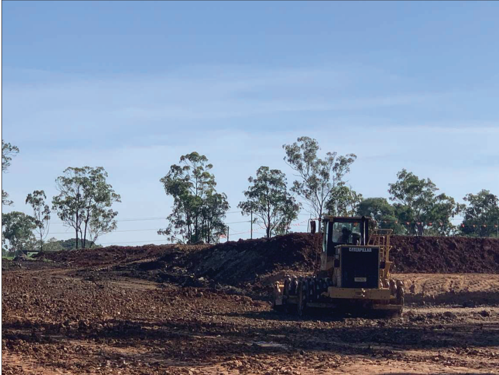
Figure 11. Compactor used throughout bulk earthworks operations. (Taken 02/03/2021)
