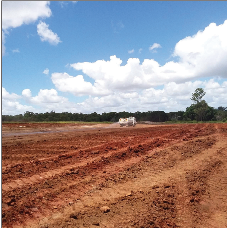
Figure 7 – Water cart applying moisture during placement of material. (Taken 15/02/2021)
