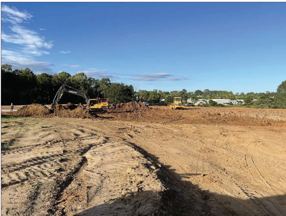
Figure 16. Excavator used throughout earthwork operations to cut and transfer material. (Taken 30/03/2021)
