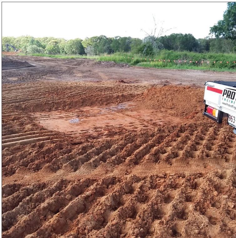
Figure 8 – Test pad cut for field density testing. (Taken 20/02/2021)
