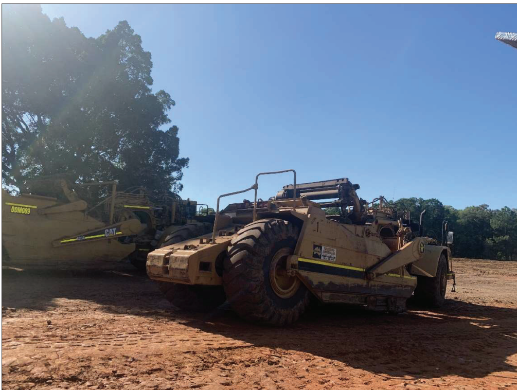
Figure 12. Scraper used throughout bulk earthworks operations. (Taken 02/03/2021)
