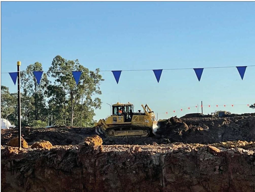
Figure 18. Dozer cutting embankment. (Taken 21/04/2021)
