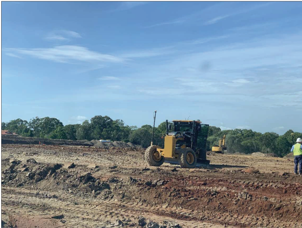
Figure 13. Grader used to trim pads throughout earthworks operations. (Taken 08/03/2021)
