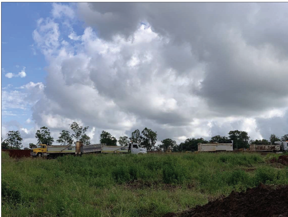
Figure 10 – Dump trucks carting fill material. (Taken 26/02/2021)
