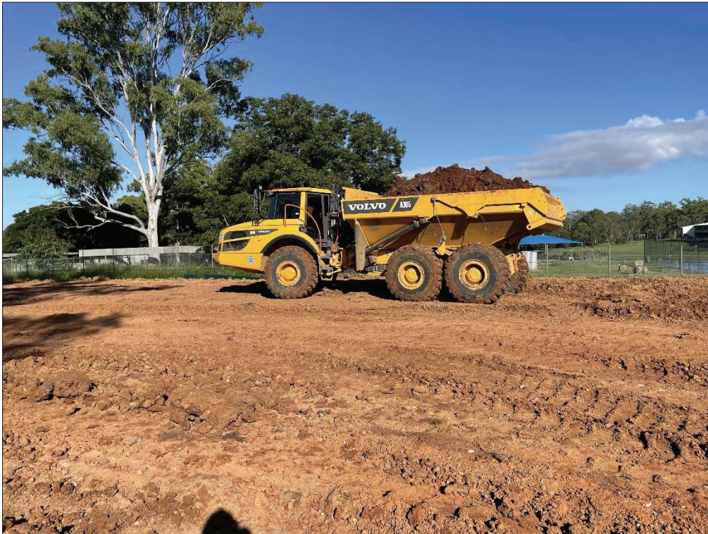
Figure 15. Dump truck transferring fill material. (Taken 29/03/2021)
